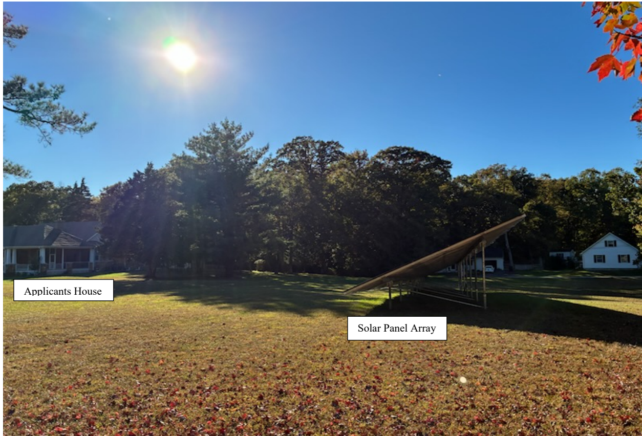
Photo No. 2 East (front) yard elevation of the applicants' house with the solar panel array to the right.
