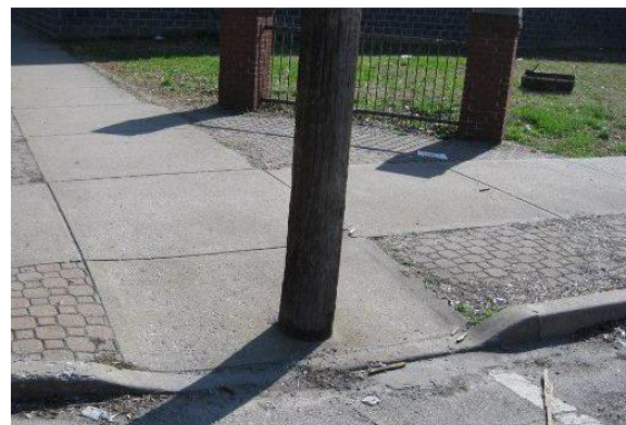
Figure 6. ADA ramp with good surface condition.
