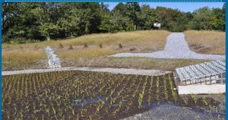
Tinkers Creek Shallow Gravel Wetland BMP Retrofit Project
