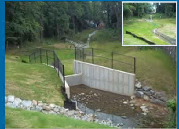
Landfare SWM Retrofit, post-construction
