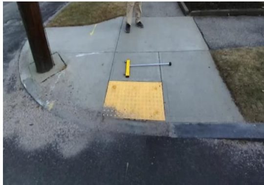
Figure 3. ADA ramp with DWS present.
