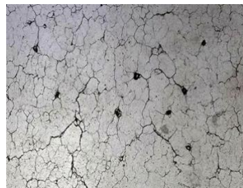
Crack 3 or severe:
