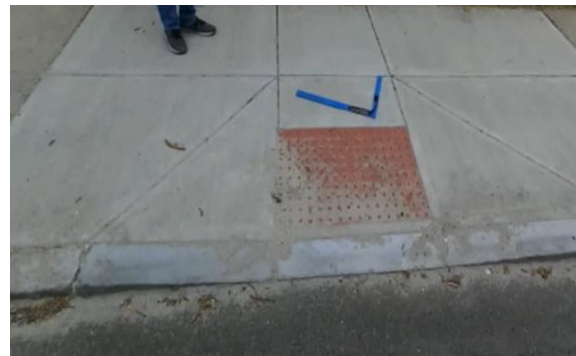
Figure 6. ADA ramp with good surface condition.
