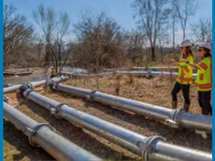
RK&K provided construction inspection services for the Herring Run Stream Restoration and Asset Protection project in Baltimore City. Rebecca Oaks and Jessica Krueger inspecting the stream bi-pass pumping.
