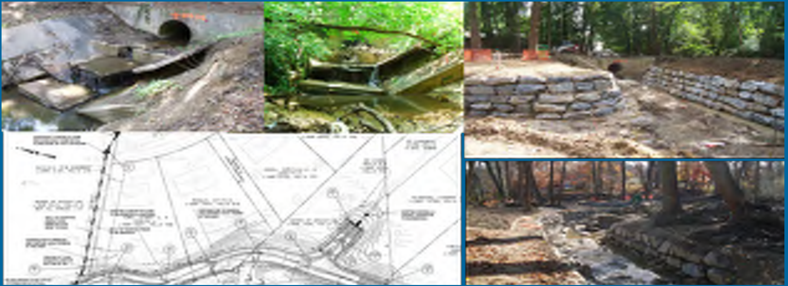
Wynnleigh Road Outfall & Stream Channel Restoration Project - Before and After
