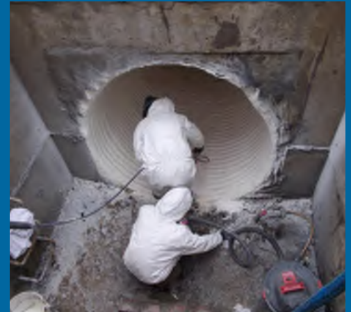
Crews at the Country Walk Culvert applying a structural epoxy coating to the storm drain inlet structure.
