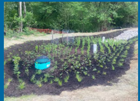
Bioretention facilities 1, 3, and 5 designed and constructed at Elk Neck State Park. These photos were taken during and right after construction completion early 2024.
