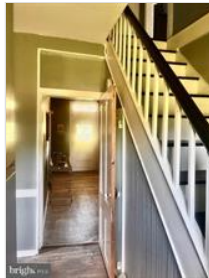
hallway and stairwell
