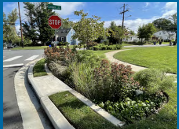
Glenmont Forest GI Facility: (L) Completed 6/2022 | (R) One year later 9/2023
