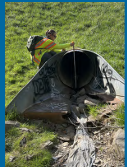
RK&K's Rebecca Oaks and Brittany Ayers Moyer performing structure verification measurements to verify PCSWMM model inputs.
