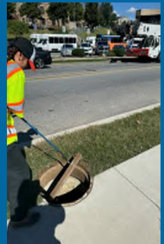
RK&K team performing storm drain inventory in Montgomery County
