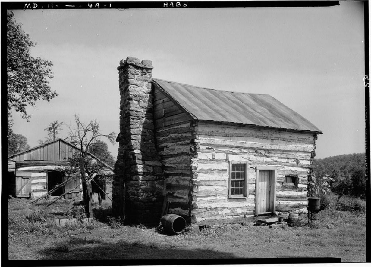
Figure 66. View of slave quarters from the southwest, Dickerson, Montgomery County, Maryland; John O. Brostrup, Photographer; September 4, 1936 ( https://cdn.loc.gov/service/pnp/habshaer/md/md0200/md0211/photos/081897pv.jpg ).
