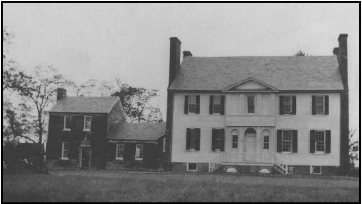
Figure 19. La Grange, ca. 1975, east façade (Rivoire and James 1975).
