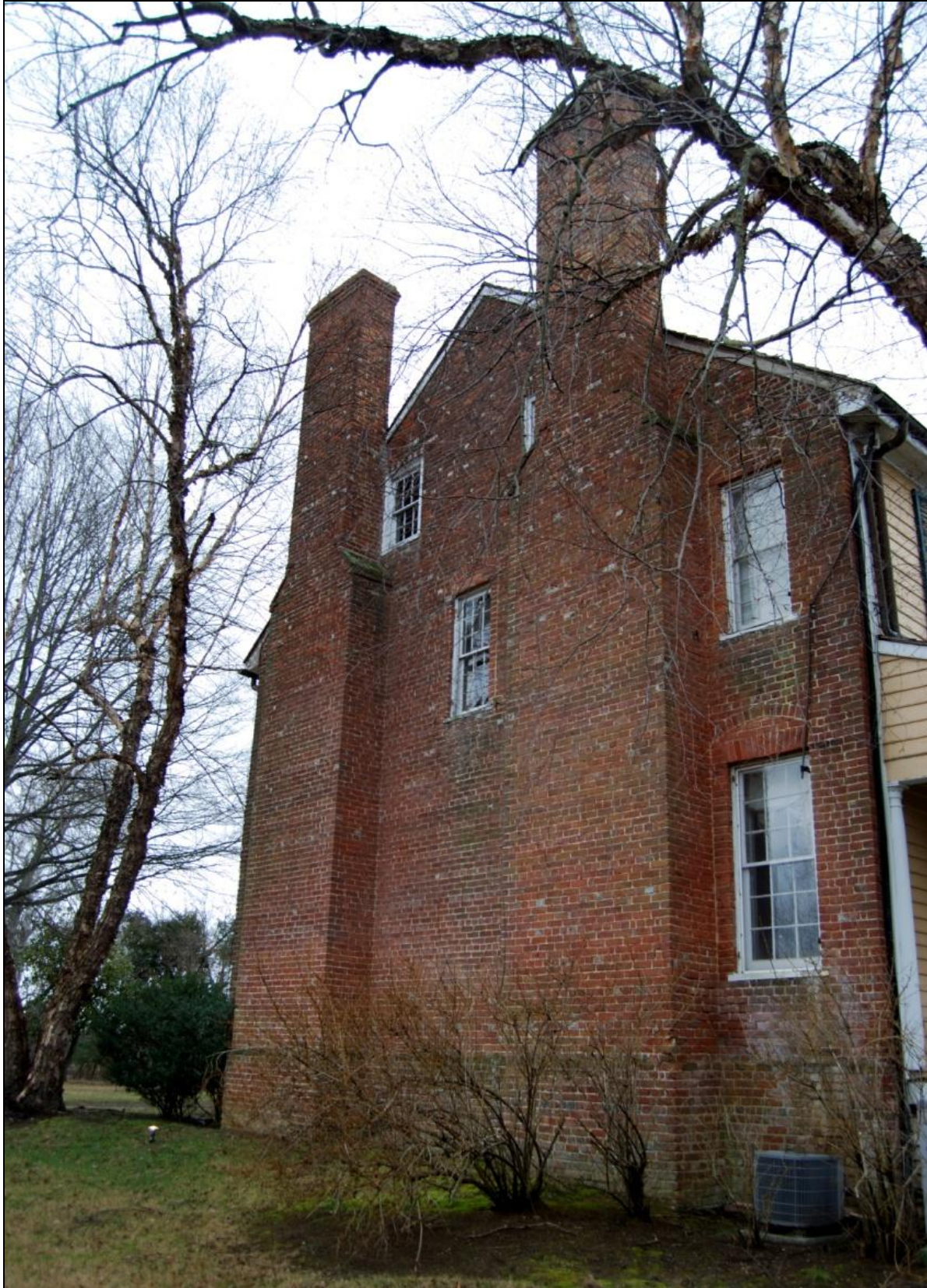
Figure 17. North gable end wall at La Grange executed in three-course American bond.
