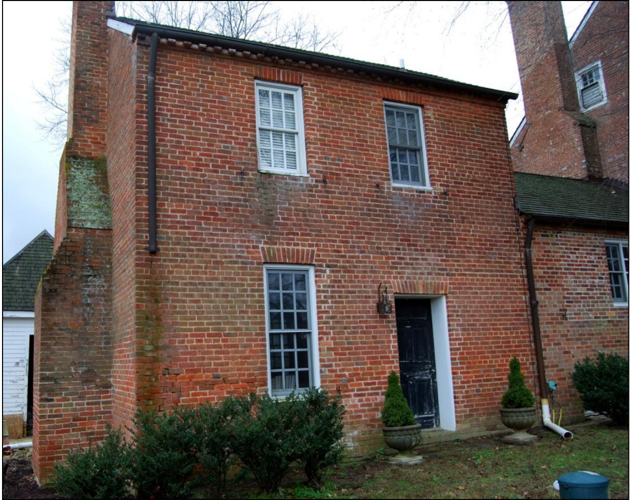
Figure 18. The two-story brick kitchen at La Grange executed in five-course American bond.
