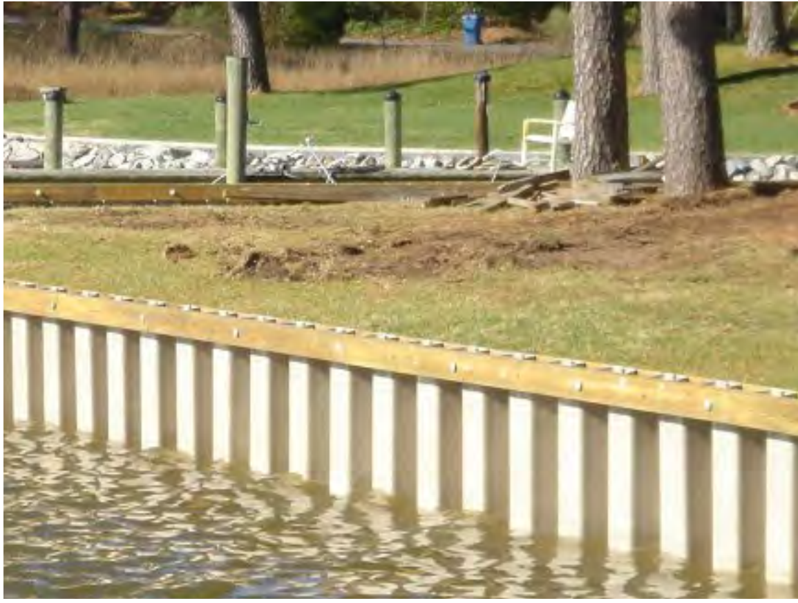
F Vinyl sheet piling along east side of the pond creates a clean edge.
